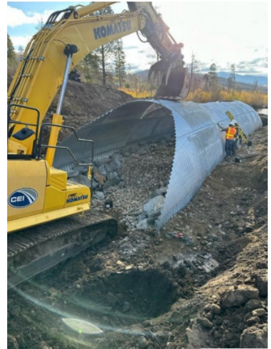
Stillwater repair construction
